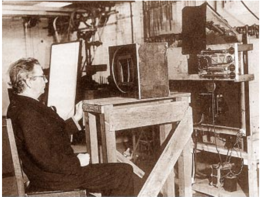
John L. Baird's 1927 3-D television using side-by-side stereo pairs
